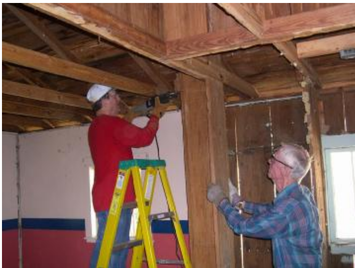
Dennis Folz and Jack Ross removing interior walls.
