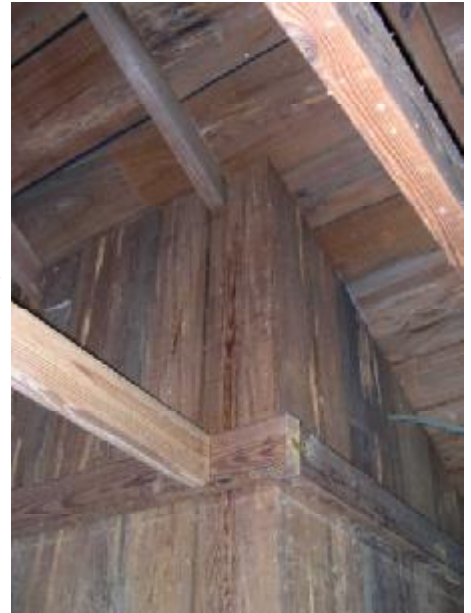
Interior walls extending to the roof.
